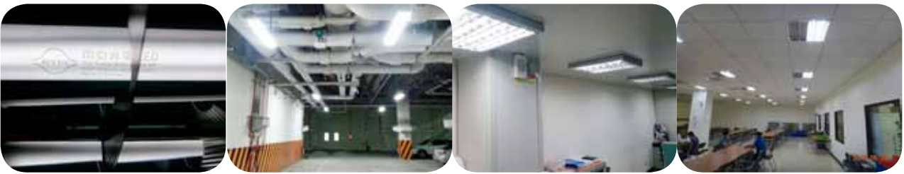
廠內燈管分區汰換為 LED 燈管
